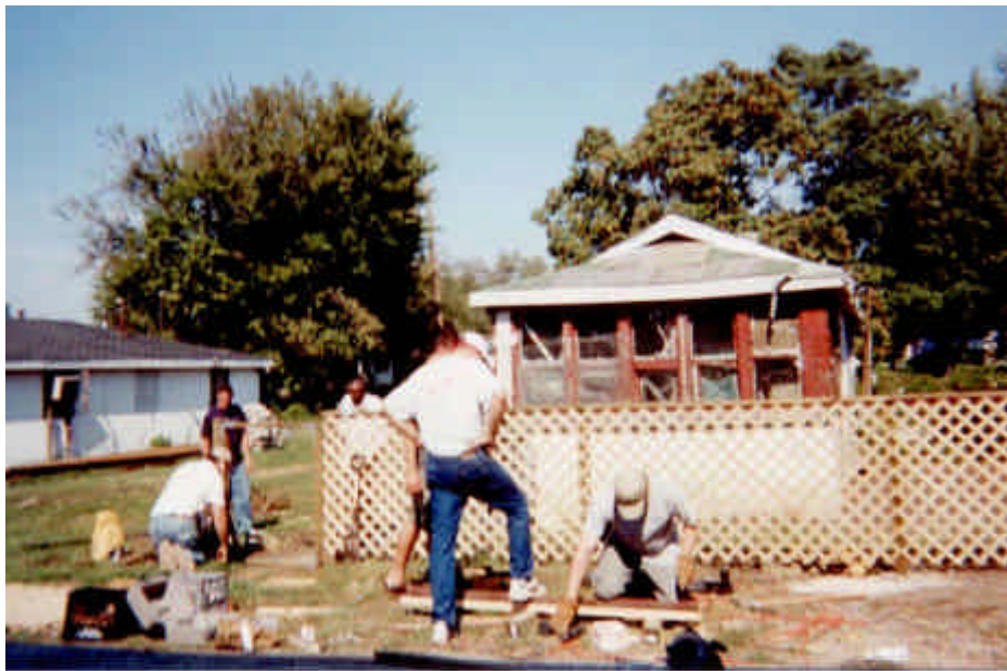
The new fence.
