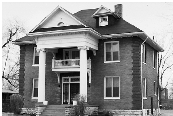
Figure 4.1. An example of housing that earned the neighborhood the nickname "Quality Hill".
