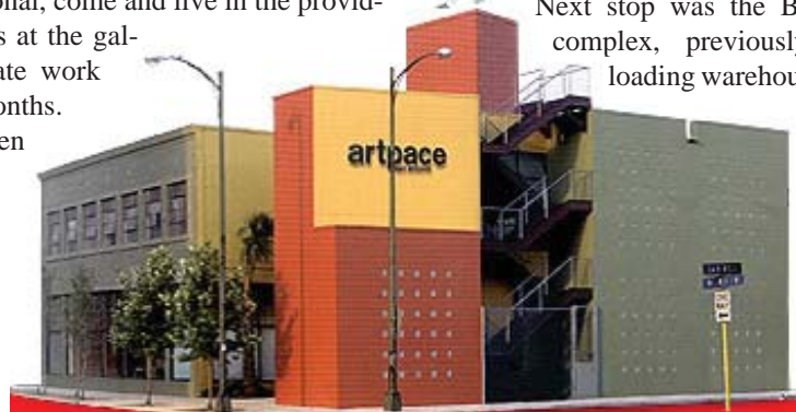
Artpace , an adaptive re-use of a San Antonio tire warehouse.
